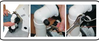
STEP 8: Install the pump header and gaskets. Then insert the temperature sensor(if applicable) into the liquid tight connector until flush and tighten.
