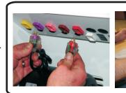
STEP 9: Plug the components into the receptacles and reinstall the lower box cover plate.
