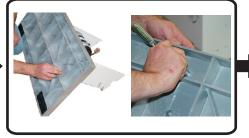
STEP 4: Flip the base with box over and install the washers and nuts. Tighten with the 7/16 deep socket/wrench.
