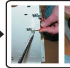
STEP 7: Use the included #8 copper wire to bond the pump to the main control box.
